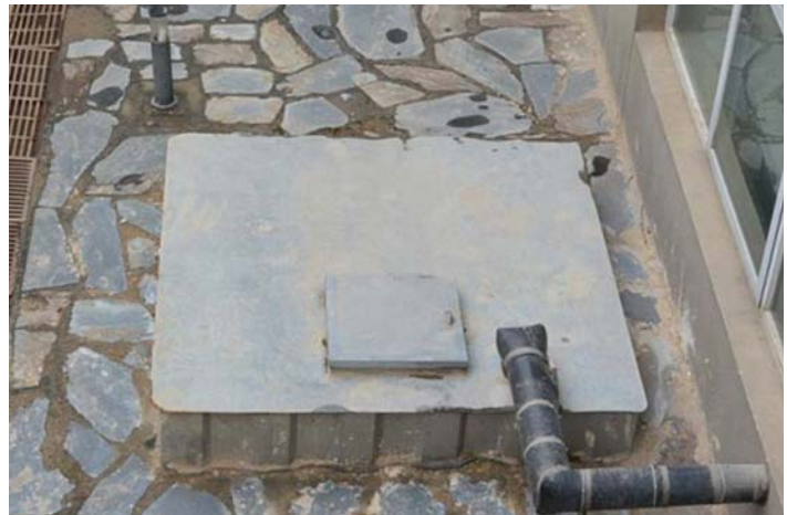
Picture 4: Recycling water tank
