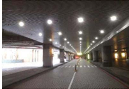
All 35W*1 driveway halogen lamps altered to 10W*1 LED ones
