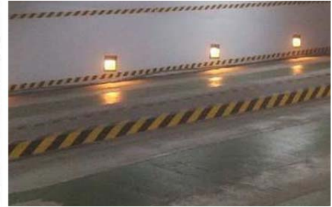
All 70W*1 driveway guide HPS lamps in B1-5 and F1 altered to 10W*1 LED ones
