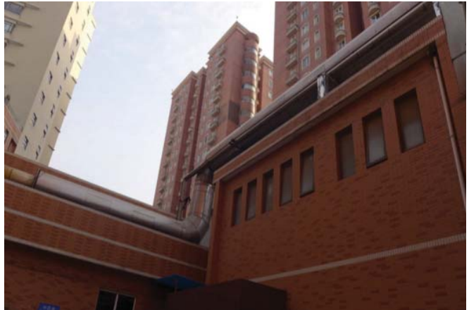
Picture 2: The boiler gas flue pipe
