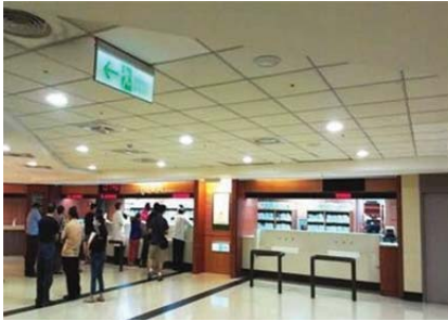
All 26W*2 PL recessed lamps altered to 12W*1 LED ones
