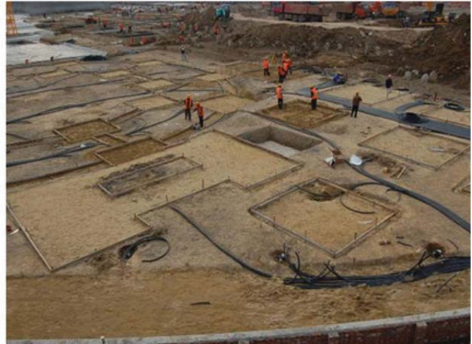
Fig6 Ground-source heat pump system-2
